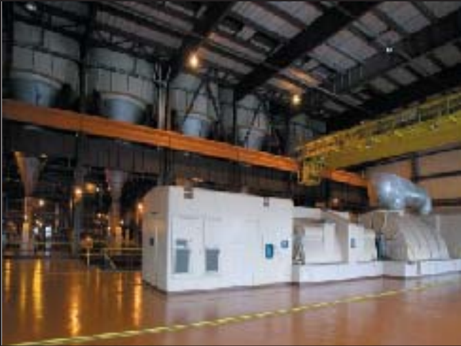
A massive turbine engine (center) generates electricity. The steam condensate return is on the right. To the left is the exciter that controls voltage and the amperage of the output.
